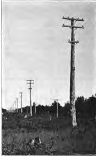
STANDARD POLE-LINE CONSTRUCTION
